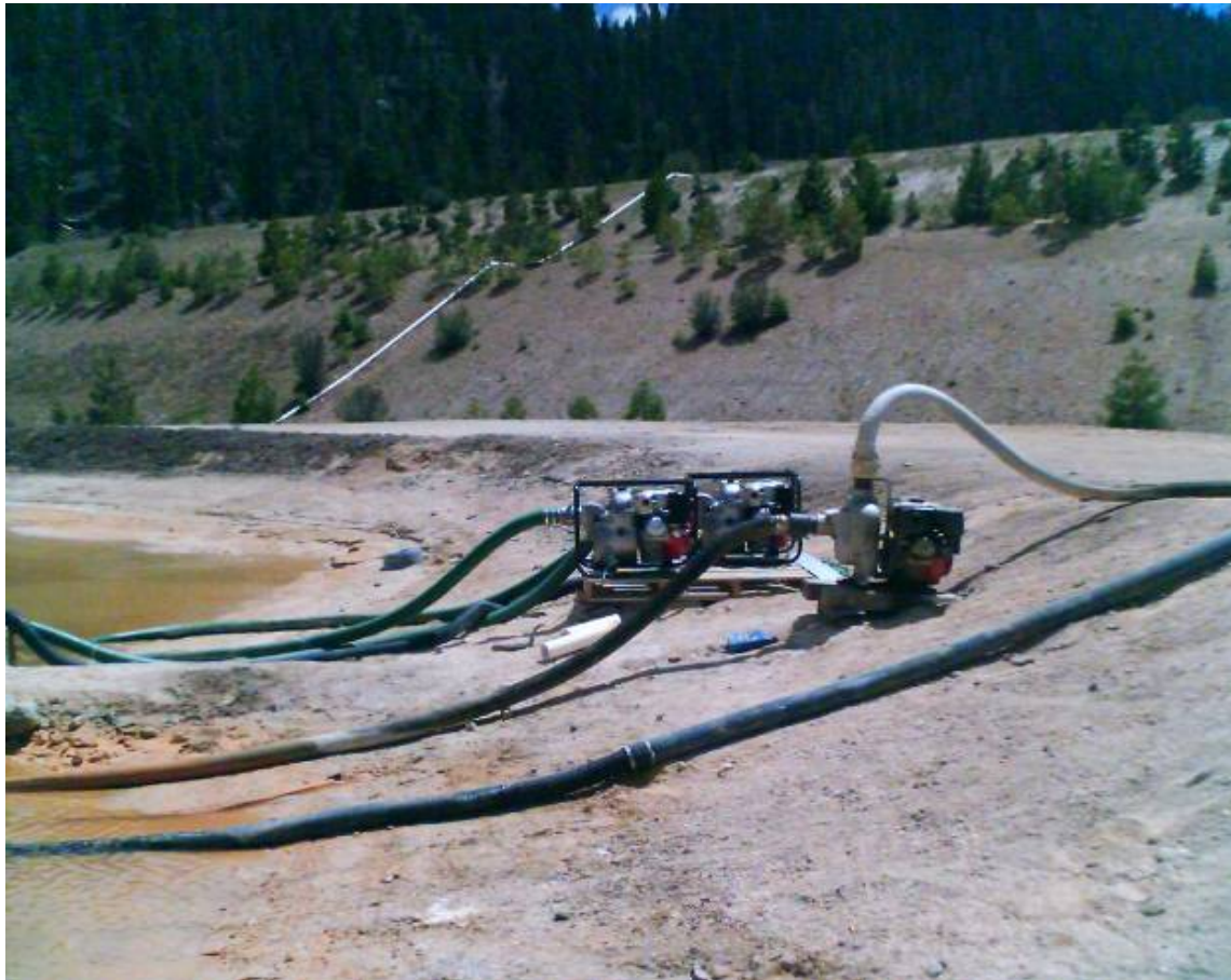
Figure 2 Water discharge from Pond 3 to the Leviathan Creek.
