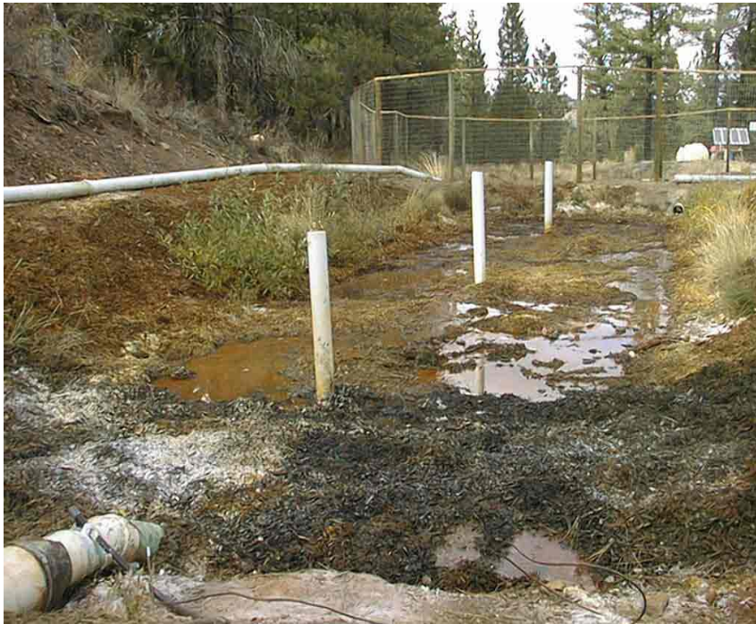
The first pond (reactor) consisted mainly of wood chips.
